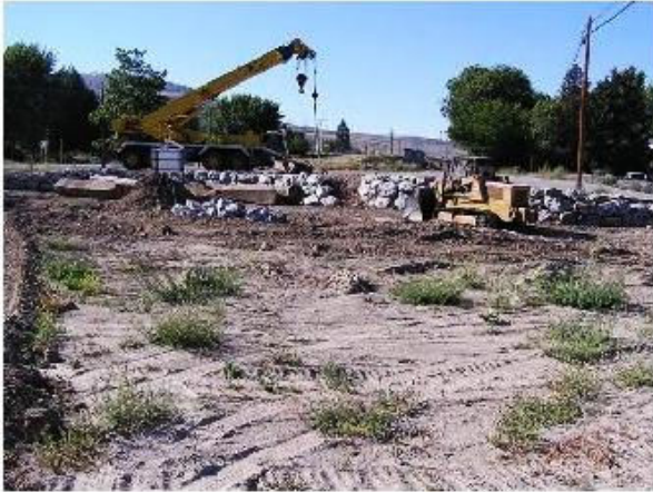
Gallup Crane Hoisting Bealt Pillars
